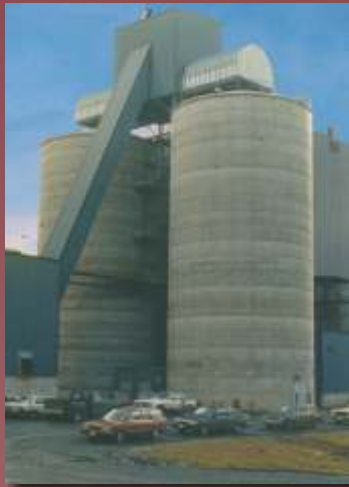
Model 698 Systems with concrete silos
