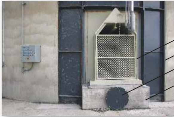
Beam Entrance Silo Frame for Beam Auger Removal Port Beam Foundation
